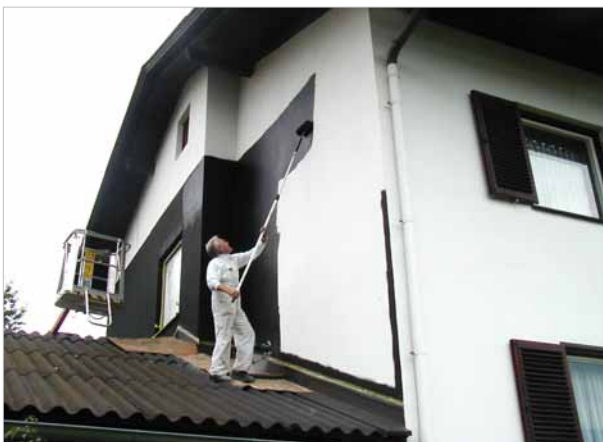
3) Grounding of the shielding paint.
